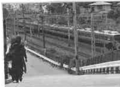
Current Ashiyagawa Tunnel
